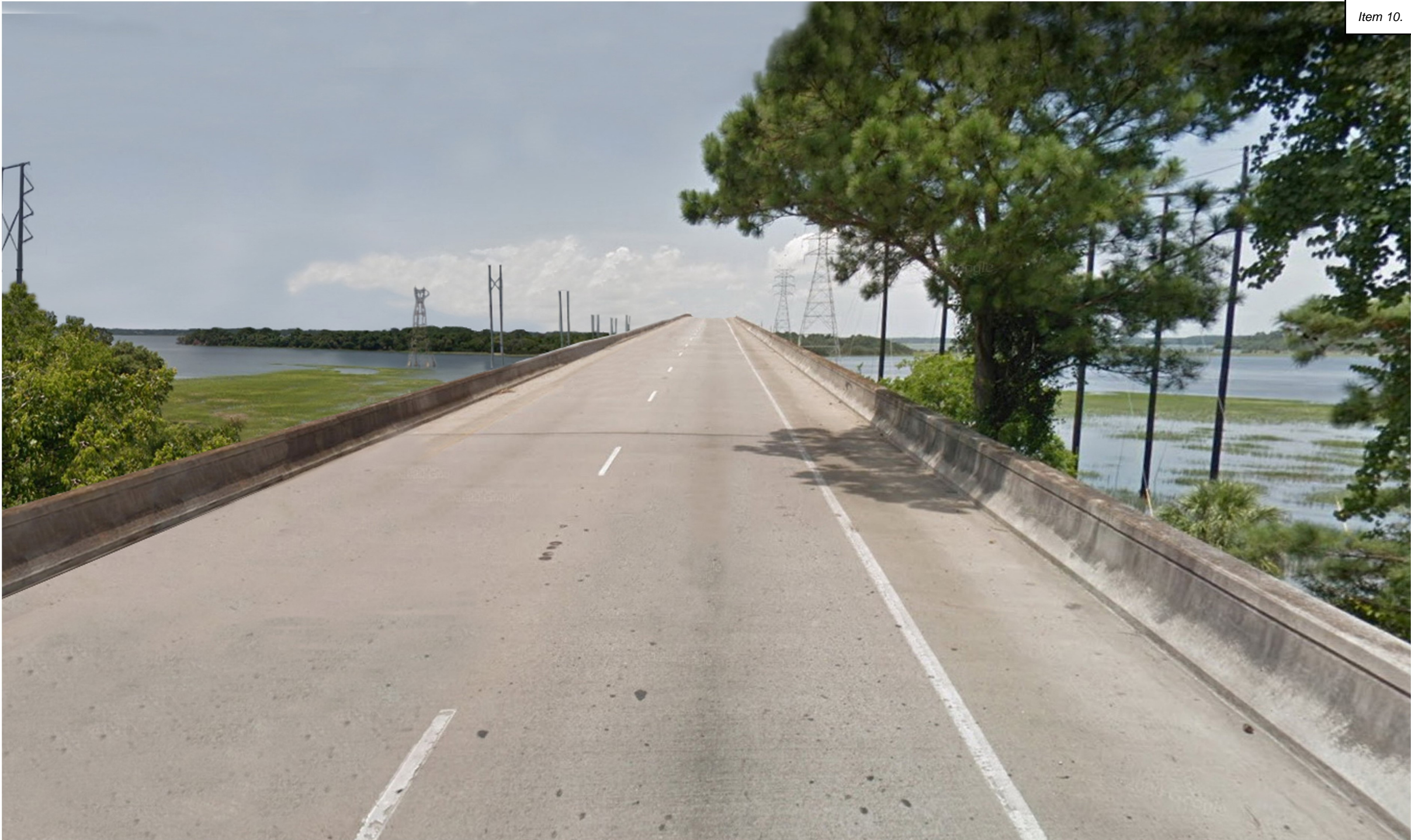
Hwy. 278 Single Bridge | Existing Conditions
