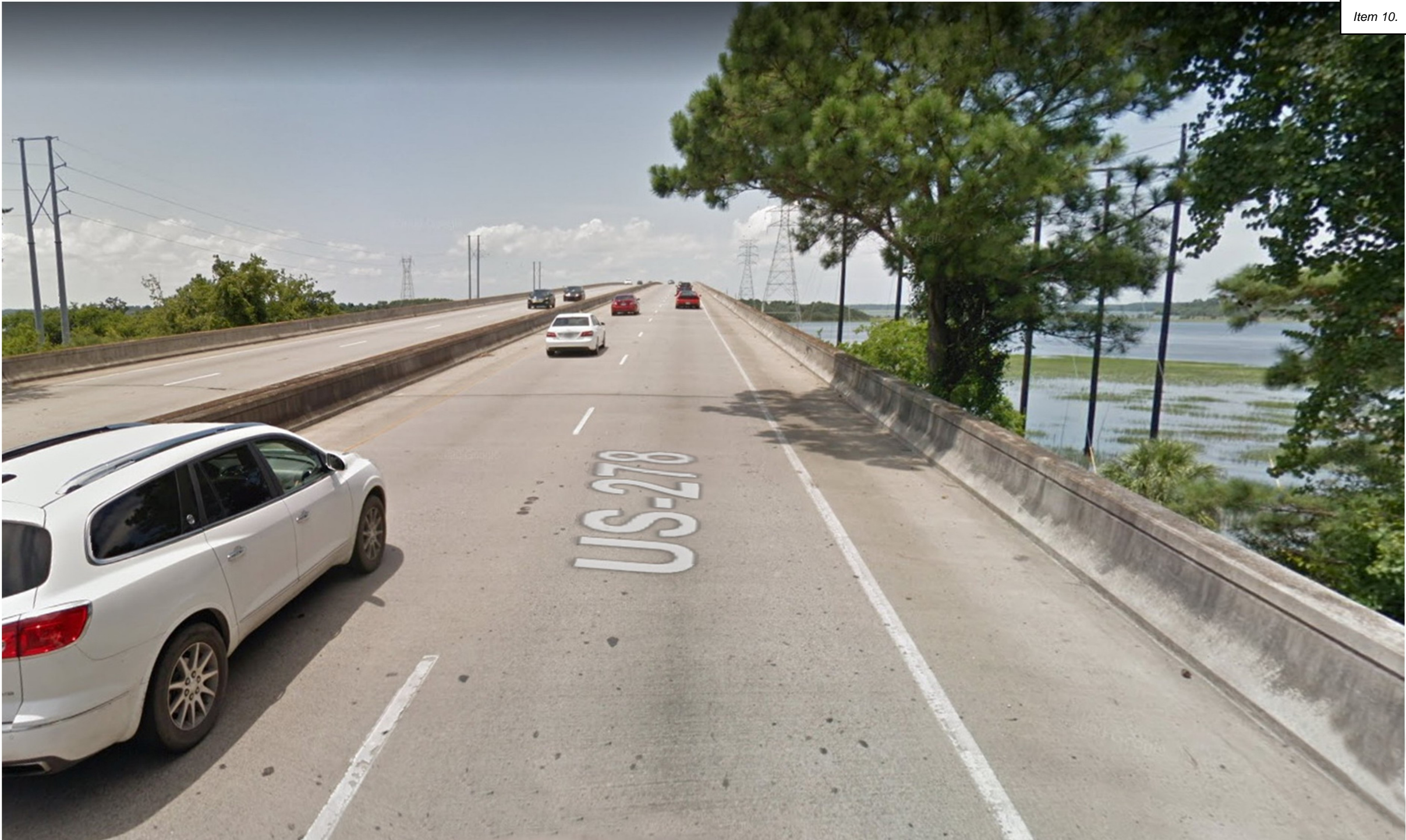
Hwy. 278 Double Bridge | Existing Conditions
